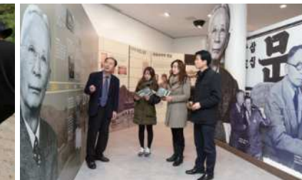
Renovation of the Seo Jae-Pil Memorial Hall
