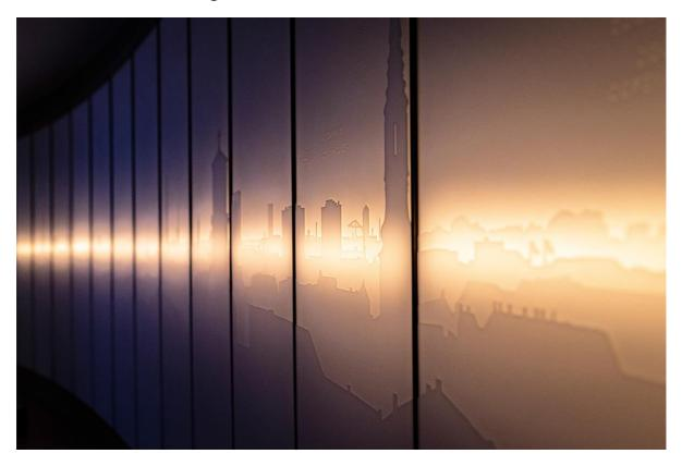
The back wall of the Museum of Copenhagen offers an impressive backdrop to the miniature model of the city. The panoramic view was milled by YOHO fabricators into the HI-MACS® material, used here in the translucent Opal shade. There are several levels of milling, which are backlit at different intensities giving an inspiring scene behind the model city.
