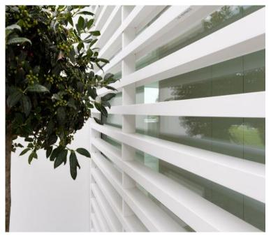
doors is flanked by two window frames which are provided with 200cm wide and 10cm deep, fixed lamellae. These provide both privacy as well as the first optical highlight made from the mineral material HI-MACS<sup>®</sup>. The 4 x 1.50 metre tall, anthracite coloured pedestals are also made from this material. Thanks to its high UV-resistance and excellent colour density, HI-MACS<sup>®</sup> is ideal for exterior use.
